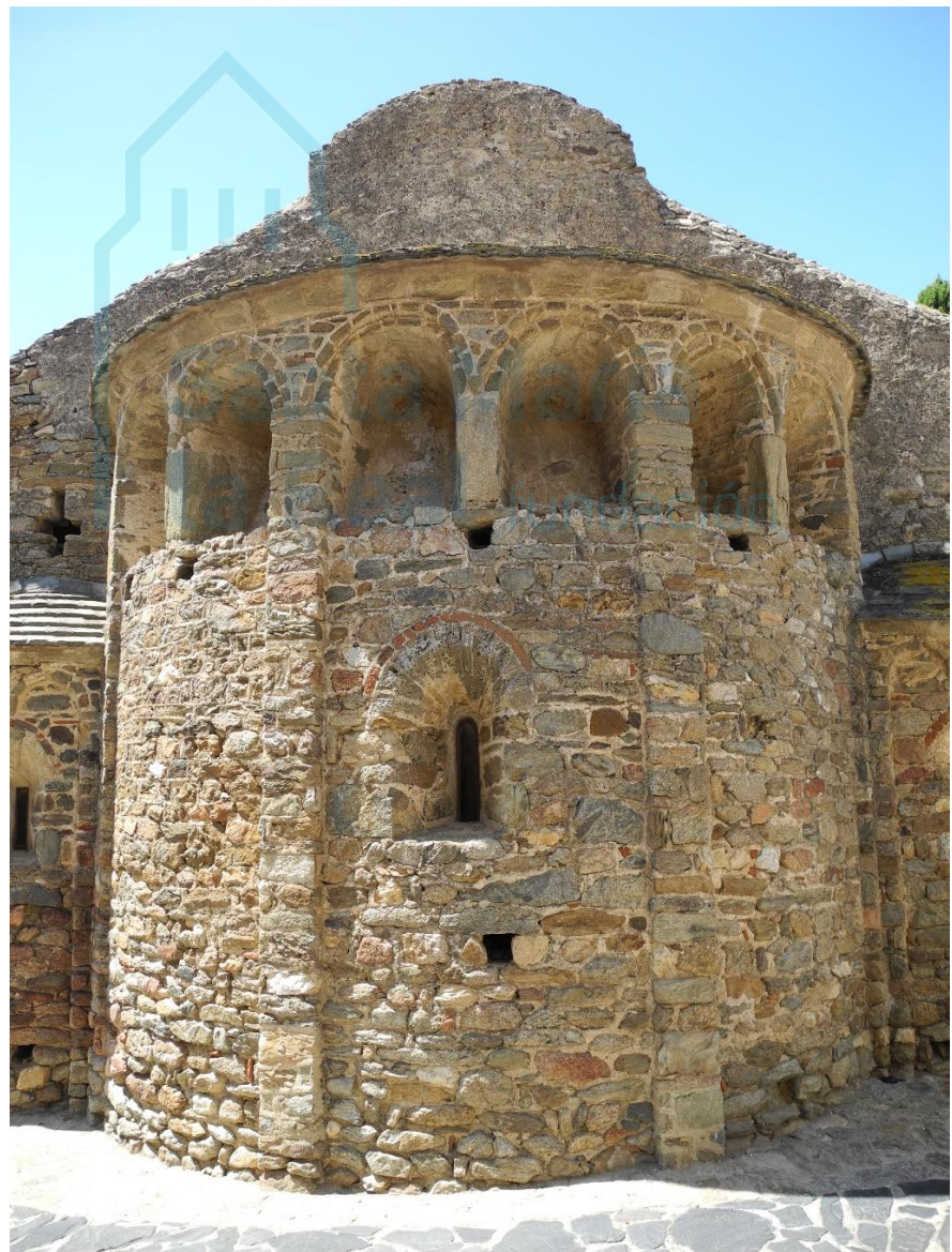
Detalle del ábside mayor
