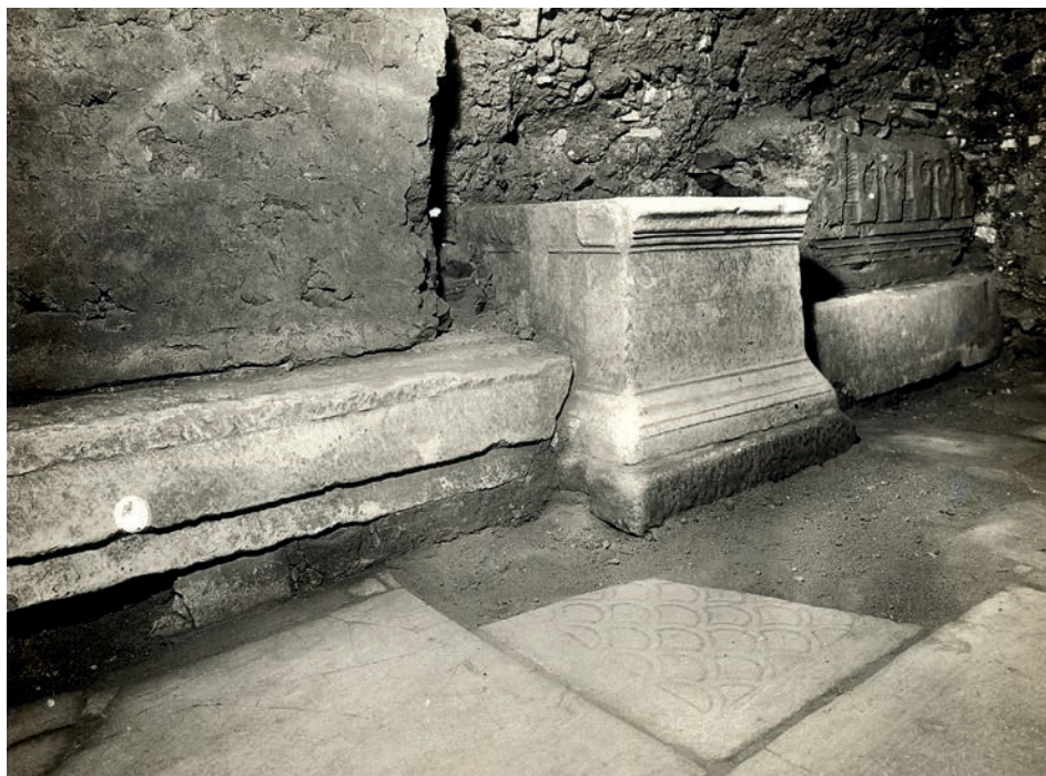
Fig. 3. St. Peter's. East face of Gregorian presbytery, south stretch with pedestal of pergula column, parapet supports and imprint of parapet slabs (left and right). Photo per gentile concessione della Fabbrica di San Pietro in Vaticano
